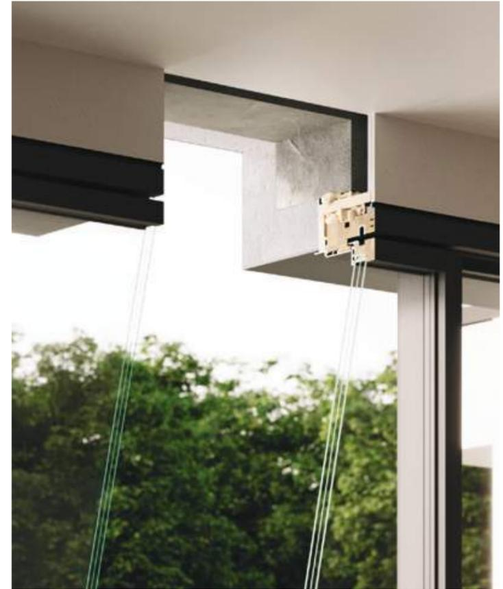
Detail of the subframe and upper sash transom of the Blend lift-and-slide sash, frame with ATF reduced trim, installed on masonry with plasterboard counterwall.
